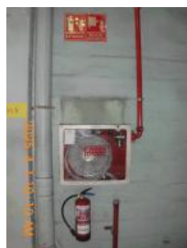
Extinguisher. Hydrant equipped with fire hose.JPG
